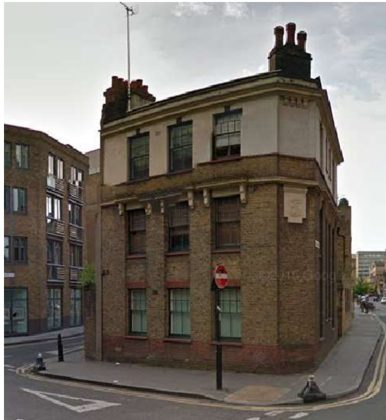
Figure 3: Existing building at No 66-68 Bell Lane
